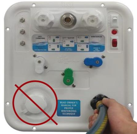
3. **FLUSH** the black holding tank(s) utilizing the tank flush line. See [Section 14L\(8\)](#) for instructions on how to flush the black tank(s).
