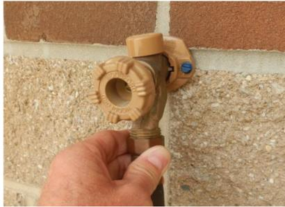
5. Fully open faucet at water supply source (40 psi minimum). Flush tank until water appears clear in 4" discharge hose.
