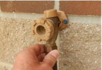
5. Fully open faucet at water supply source (40 psi minimum, 275.8 kPa). Flush tank until water appears clear in 4" (10.16 cm) discharge hose.
