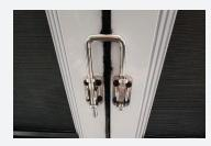
2. Rotate the lock and allow it to fall.
