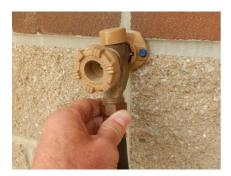
4. Turn water supply on at source. Fresh water tank should begin to fill.
