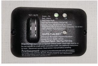
THE CO AND PROPANE GAS ALARM. SEE <u>SECTION 4G</u> FOR ITS LOCATION IN THE RV.
