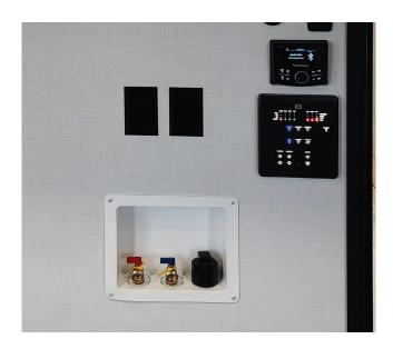
Because there is no exhaust for the dryer in the garage, if installed in this location, a ventless dryer MUST be used.
