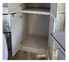
The clothes hanging rods and the shelves in this cabinet are removable to permit installation of the washer/dryer. Upon installation both will need to be fully removed. Below is a photo of the water connections in the master bedroom.
