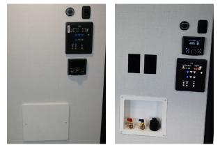
Because there is no exhaust for the dryer in the garage, if installed in this location, a vent-less dryer MUST be used. Please contact your Dealer or appliance manufacturer for additional information and installation assistance.
