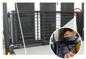
4. Starting with the first outermost section of the patio rail kit, carefully swing the rail towards the edge of the ramp door.
