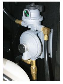
After the LP cylinder is refilled, remember to reconnect the pigtail line and secure the LP cylinder with the provided straps. If you would like notice before the regulator begins to pull from this cylinder, leave the valve closed. This will prevent the regulator from switching to the opposing LP cylinder without notice.
