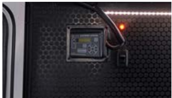
Red Light ON = Flip-Up Countertop isn't pushed in.
